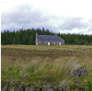
The Croft House now serves as a bothy
